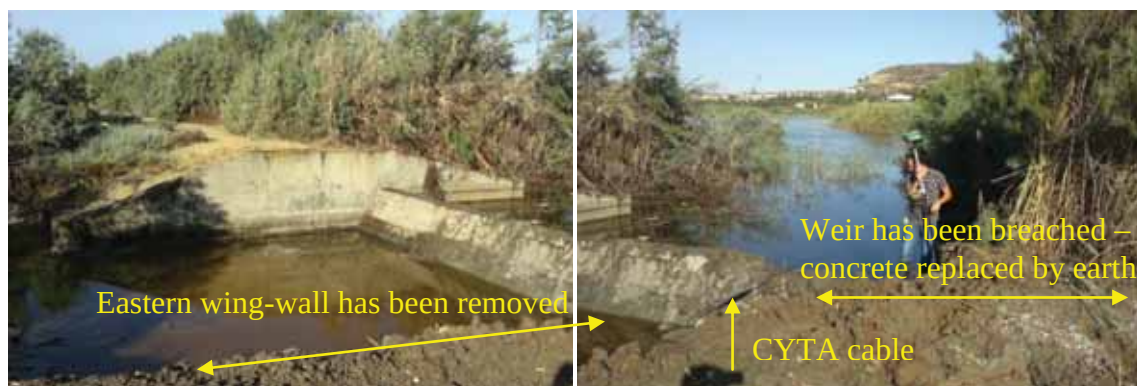
Photo 17: Conditions at the Weir on the 10 th October 2012, West view (Left) and north-west view (Right)
