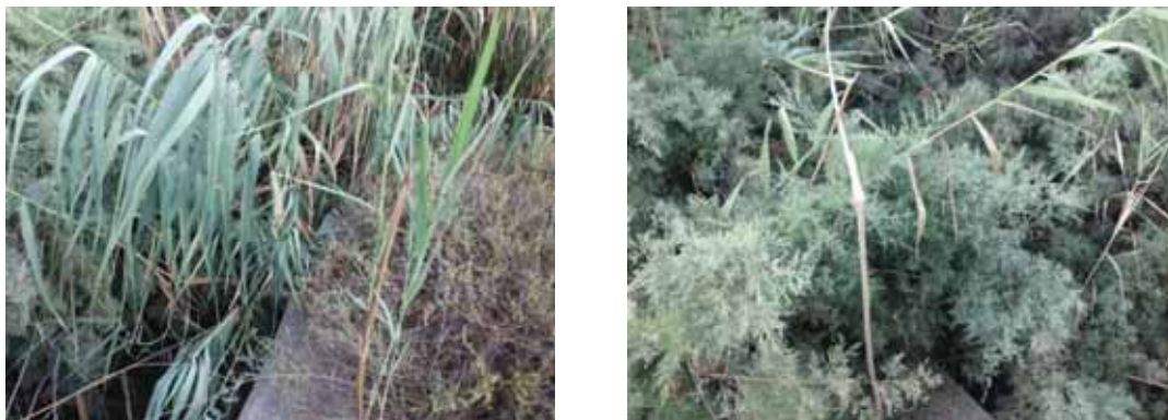
Photo 11: Conditions at the Weir on 16 th August 2012, South view (Left) and same area, North view (Right)
