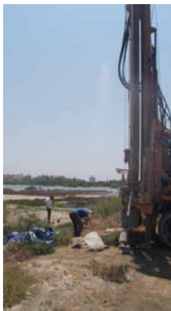
Photo 1: Drilling at the lake
