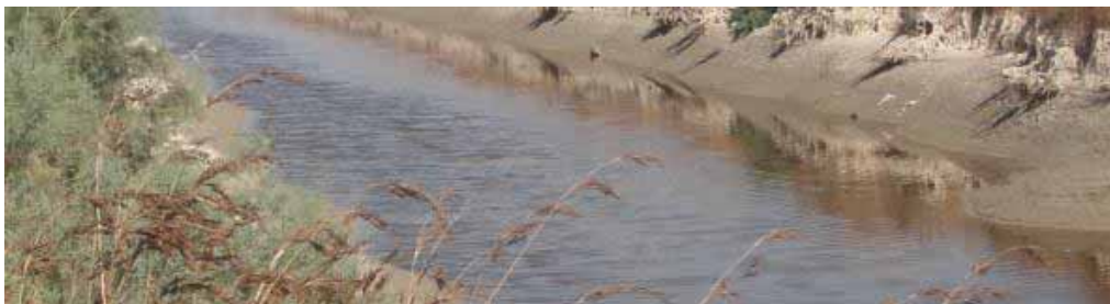
Photo 19: Sections of the North –south main channel showing characteristics of the geometry and protection of the slopes.
