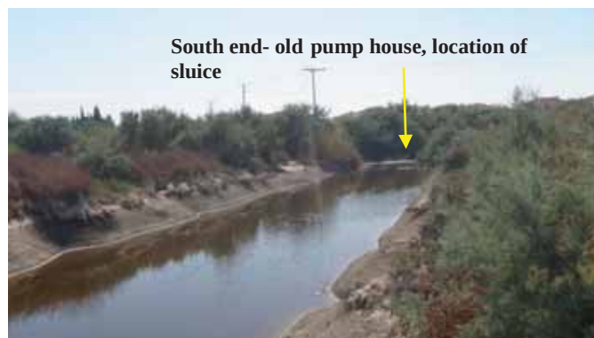
Photo 20: The main north-south ditch and the south end at which the sluice could be installed
