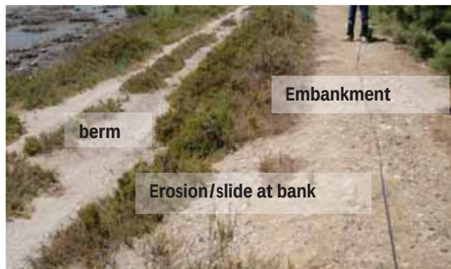
Photo 13: Photo 3: Burrows and anthills at 45m from western most point on embankment (Left) and erosion/slide at 75m (Right)
