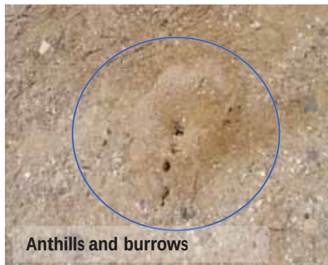
Photo 13: Photo 3: Burrows and anthills at 45m from western most point on embankment (Left) and erosion/slide at 75m (Right)
