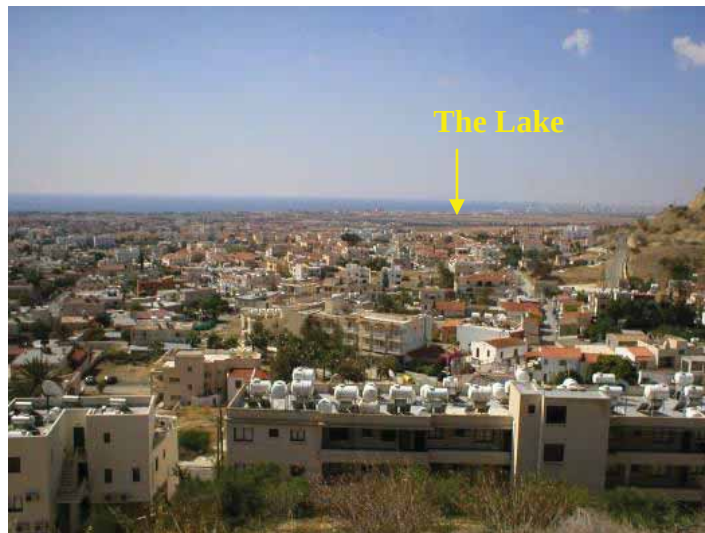
Photo 18: The urbanized area of the runoff catchment (68% of the total)
